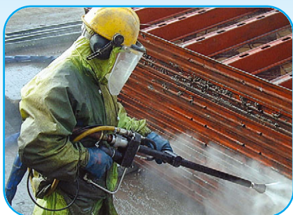
Single gun surface preparation
