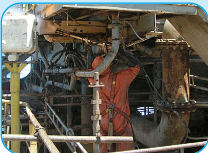
Offshore surface preparation aboard a jack up rig
