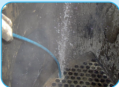
Heat exchanger cleaning - 33 lpm / 800 bar
