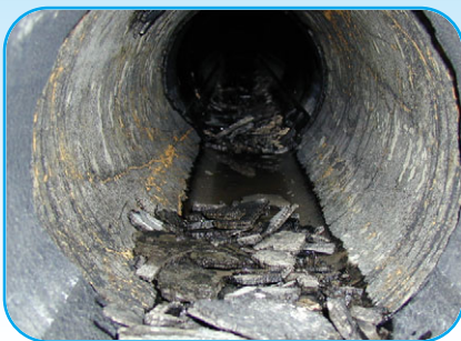
Descaling large diameter pipework – 200 lpm / 1000 bar
