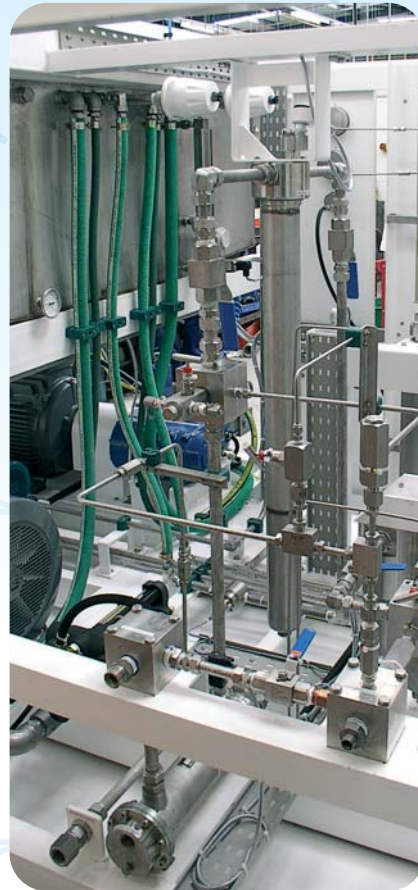
Twin HP5650 glycol pumps, flushing & pressure testing subsea umbilicals
